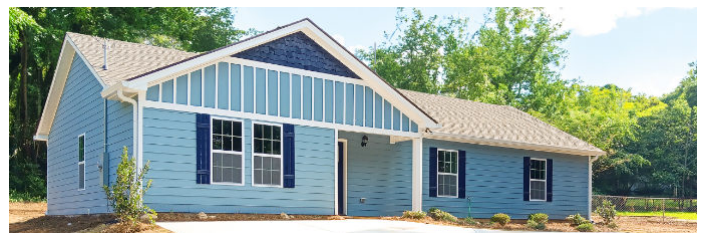
Margaret's newly constructed Habitat Home in Monroe, Georgia.
